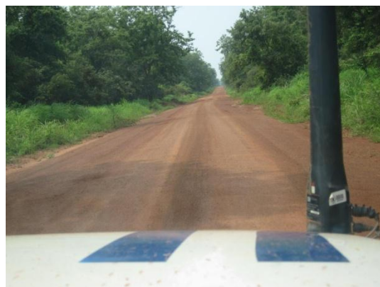
AB. Rumbek to Wullu Road
