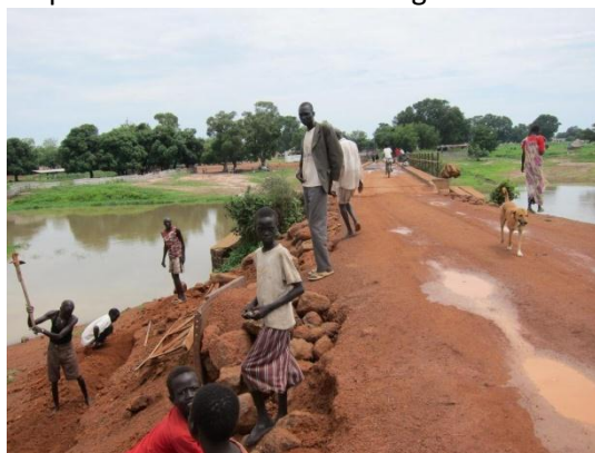
Z. Ton Bridge access Road
