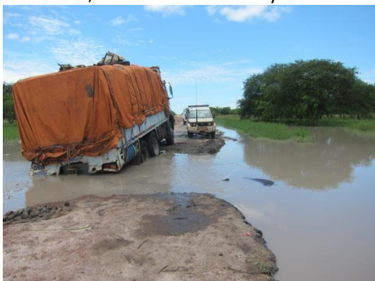
O. Rupkuai culvert road eroded (2 Sep 2012)
