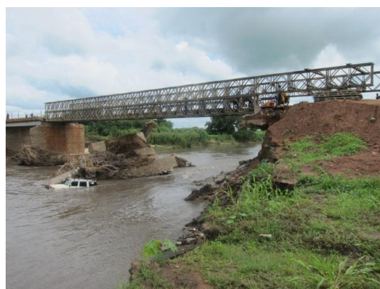
AE: Luri Bialy Bridge installed on 26 June 2012 (after)
