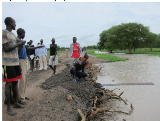
P. Rupkuai culvert repaired by local community (11 July 2013)
